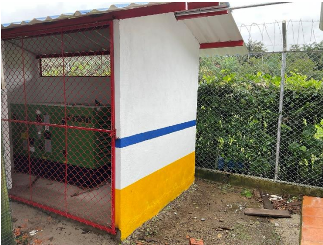
Progress at the Camp
